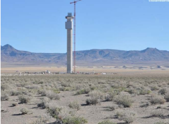
The nearly completed tower
